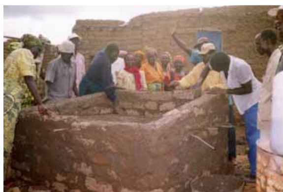
Participants at a training workshop construct a Chorkor oven in Apibase (Chad)
