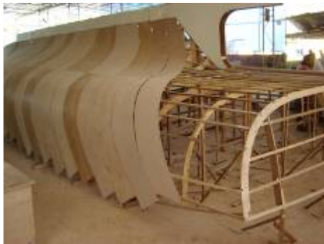
Plug under construction
