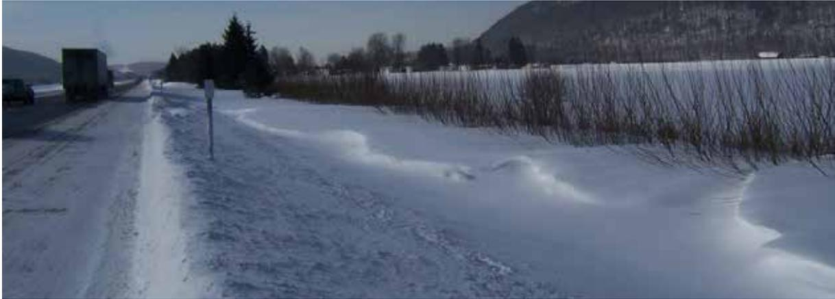
**Fig.2:** A SWLSF planted along an interstate highway in New York with at a setback distance of just 10 m and a seasonal downwind snowdrift fully contained within the setback distance between the fence and the road.
