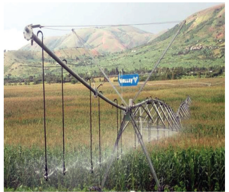
An irrigation facility in Muvumba.
