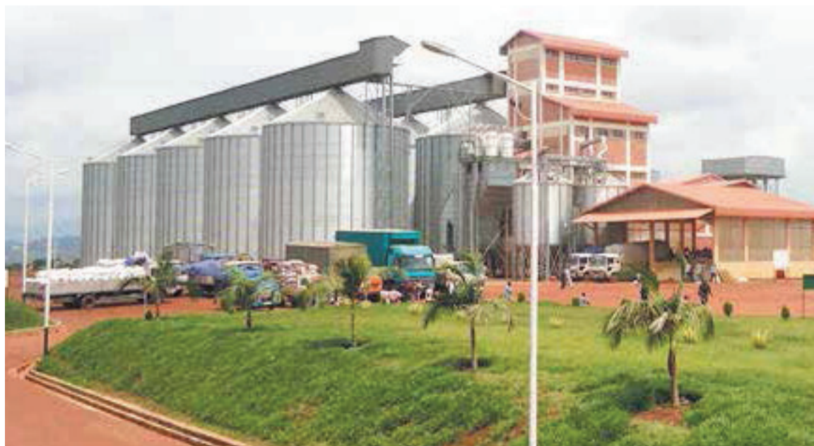
Storage facilities for National Strategic Reserves in the Kigali Economic Zone.
