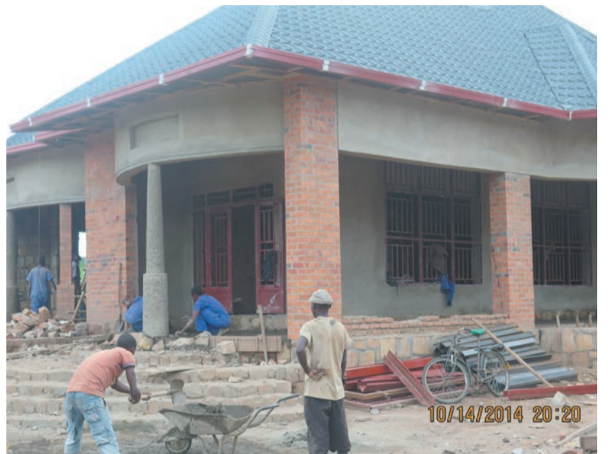
Copropriz guest canteen under final stages of construction
