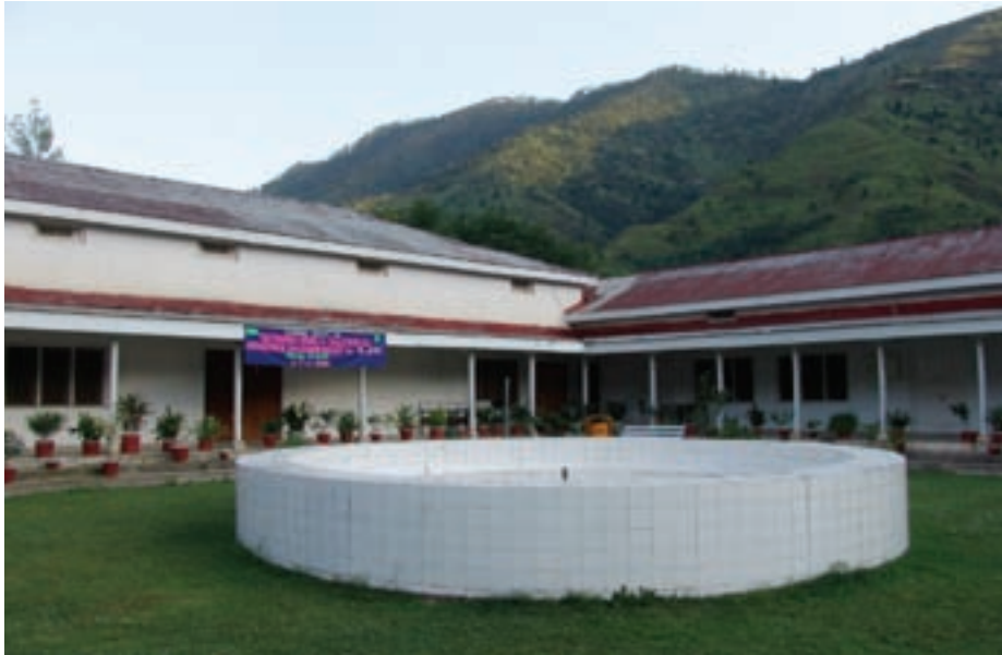
A picture of the Extension Services Management Academy taken on the occasion of a capacity building workshop on natural resources management in 2004. This building was destroyed in the October 2005 earthquake (Obaidullah Kehar)
