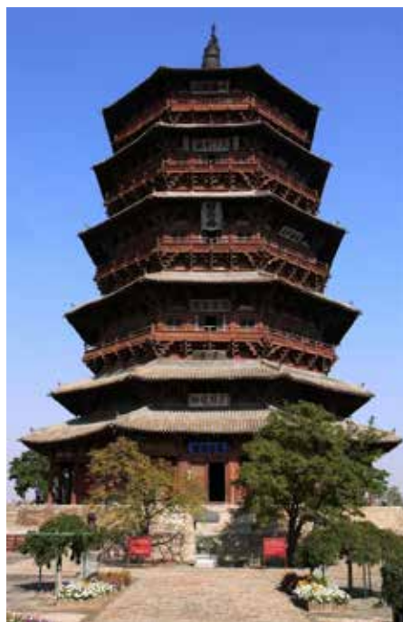
The 67 m high, nine-storey wooden pagoda of Yingxian County in Shanxi Province, China, completed in 1056, is one of the world's oldest standing multi-storey wooden structures
