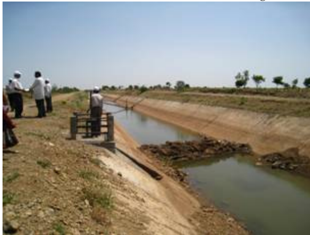
Plate 3. Rudimentary Cross-regulator built by farmers to raise water head in ALBC
