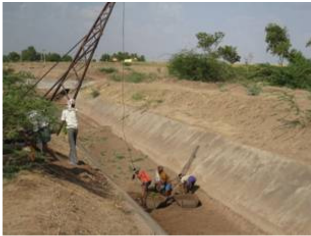
Plate 8. On going desiltation works.
