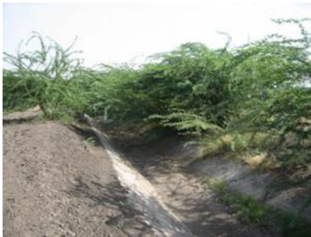
Plate 5. Secondary canal in ALBC, jungle limiting access.
