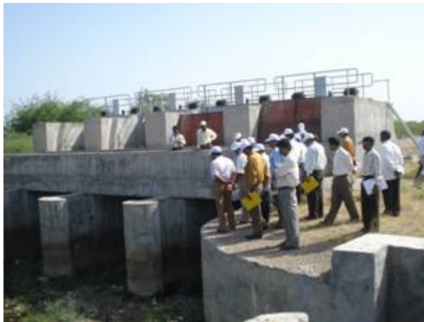
Plate 2. Cross-regulator use to channel out excess water through near by escape ALBC
