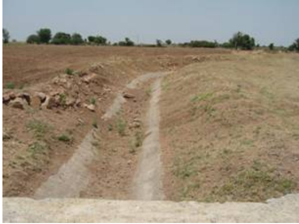
Plate 7. Secondary canal at tail end of ALBC, section largely reduced by depot.
