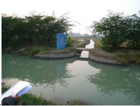
Plate 6. Golahi Minor Offtek on Nagapur Dy. @ KM 32.02
