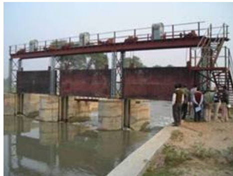
Plate 8. Low sensitive CR 44.26 KM: Overshot [gates opened, head on crest = 1meter S= 0.50]
