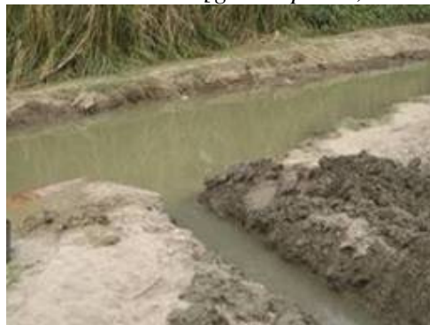
Plate 9. Typical offtake along a minor serving a field channel highly sensitive to variation of water level S=6 Detailed calculations are given in table 8.
