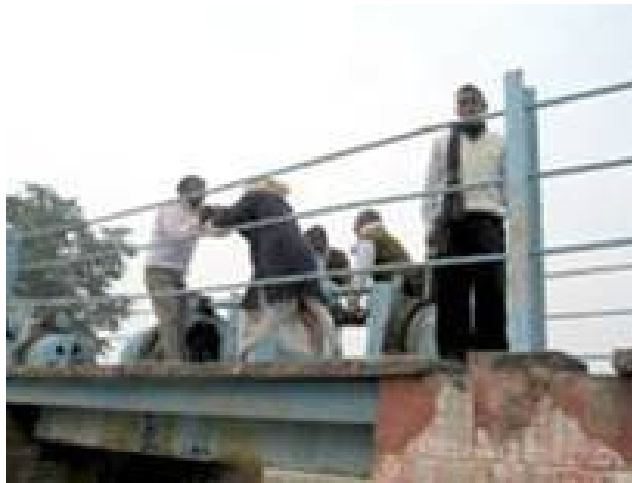
Plate 5. A difficult to operate cross-regulator along JBC: 4 people required for gate setting.
