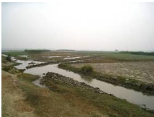
Plate 7. Tail end of Shivgadh minor of Jaunpur Dy. Lack of control structure
