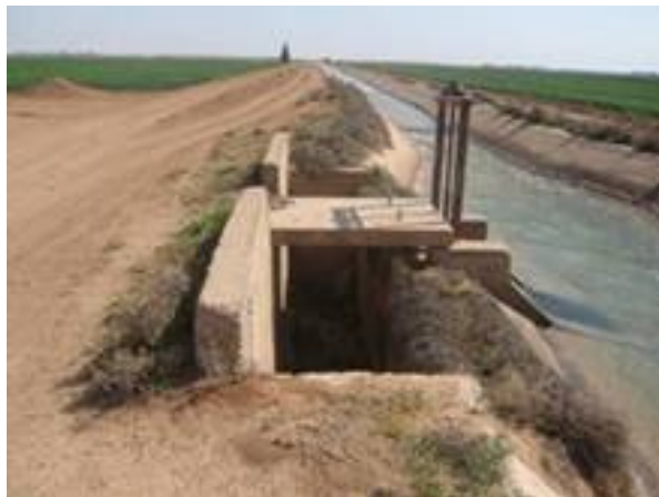
Plate 4: Spill along tertiary canal (lateral weir on the side of the offtake spilling in the quaternary channel).
