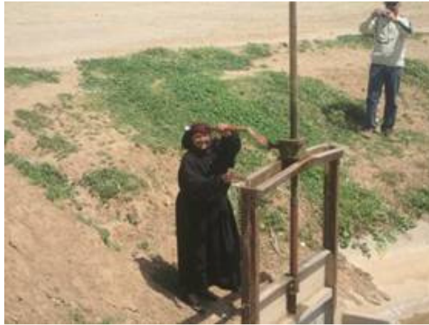
Plate 5: Gate operator moving the gate of a tertiary canal
