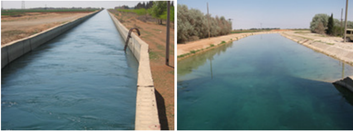
Plate 2: Main canals: Rectangular section (left) and trapezoidal section (right)
