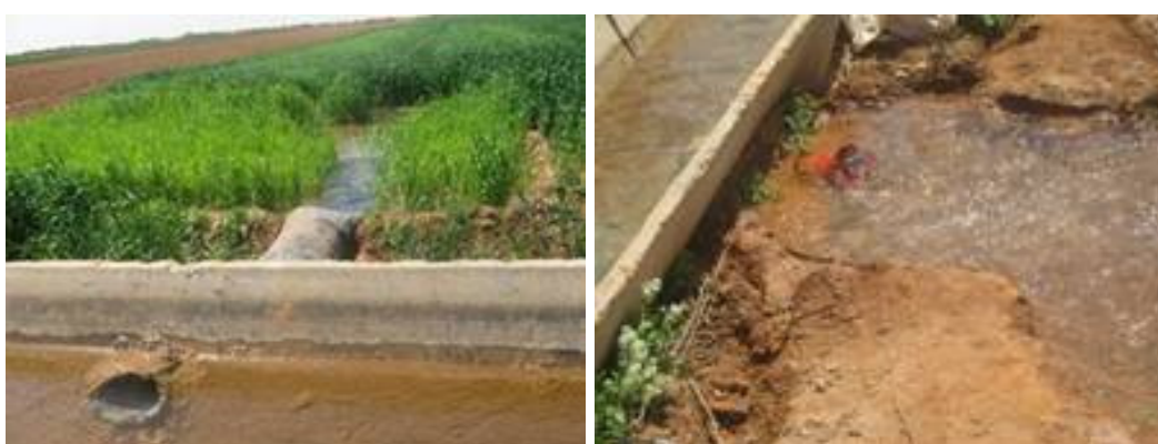
Plate 7: Illegal offtakes from quaternary canals
