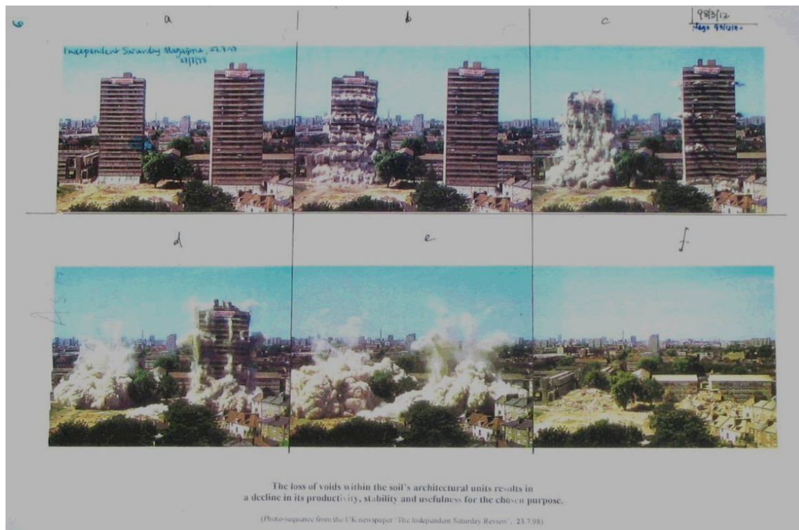
Figure 6: Controlled demolition of twin apartment-blocks. The interesting things happen in the spaces of soil architecture, as in a building. If the spaces are lost, the usefulness is lost, even though the physical parts remain.
