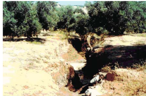
Plate 4 Another example of rill and gully erosion in a Portuguese olive orchard
